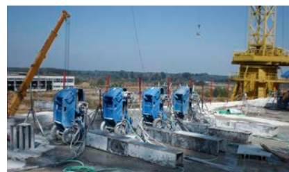
3 BULGARIA, Belene Decommissioning of a nuclear power plant
