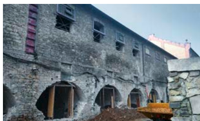
2 GERMANY, Würzburg Renovation of Bürgerbräu
